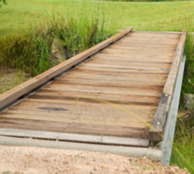
Timber Decking Bridge Spotted Gum
