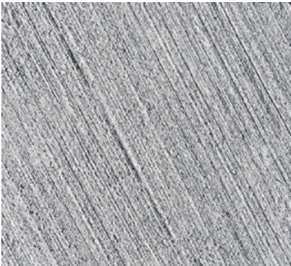
Concrete Paving 01 Broom finish concrete
