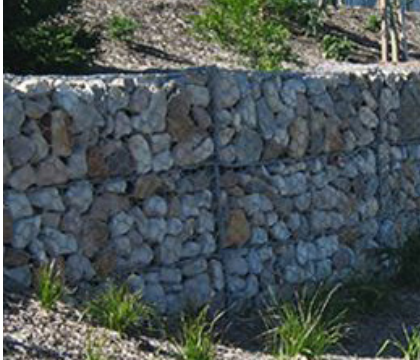
Retaining Wall Gabion wall
